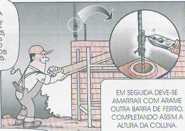
EM SEGUIDA DEVE-SE AMARRAR COM ARAME OUTRA BARRA DE FERRO, COMPLETANDO ASSIM A ALTURA DA COLUNA.
